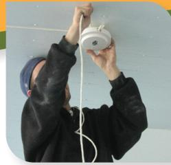
By comparison, sound masking components are small and the installation process tidy. They can typically be installed without conduit in most jurisdictions. The work can be handled discretely after hours or with only minor disruption to occupants during regular hours. There are few requirements for power tools, making the work relatively quiet, and unless the ceiling is unusually high, only ladders are needed to gain access.
